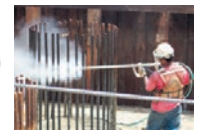
Removing rust from rebar in bridge piling.
